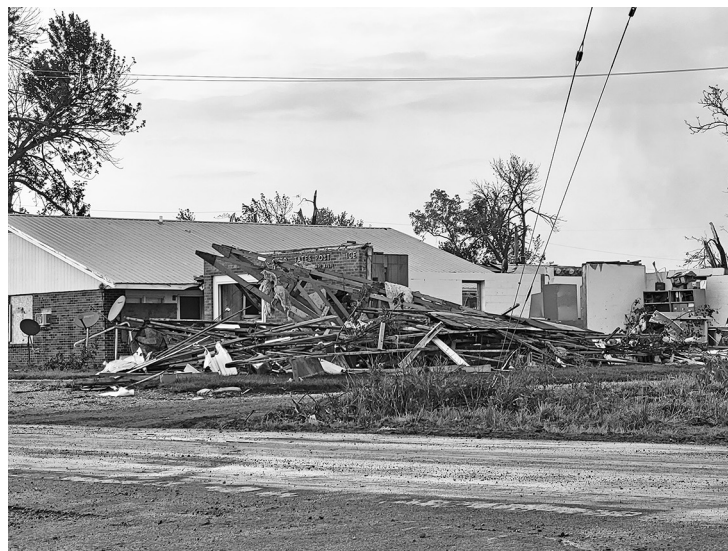
TOP: Sunlight breaks through rain clouds over homes that were devastated by an EF-2 tornado in Baring. BOTTOM: The Baring Post Office stands in ruin following the Aug. 4 tornado. — Photos by Jay Nies
